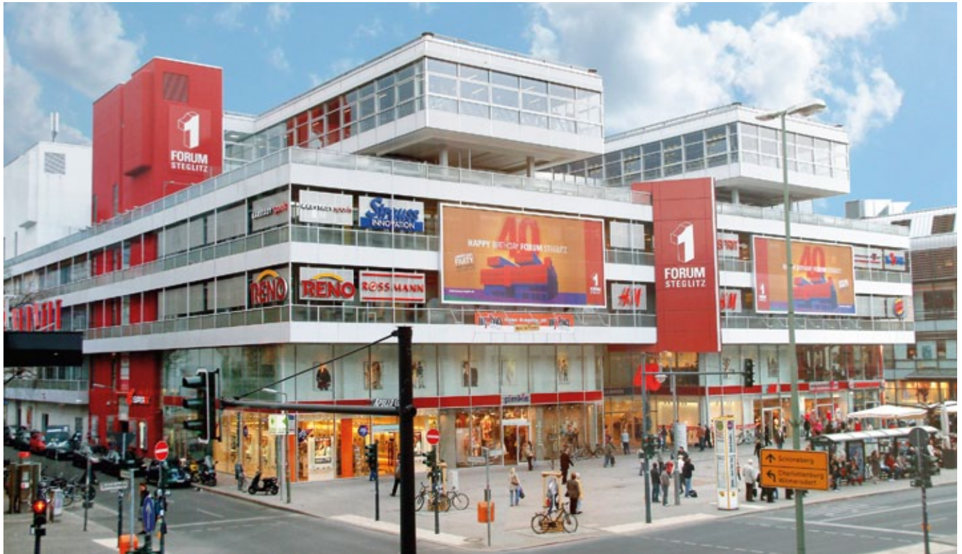
▲ Refurbishment geglückt: Forum Steglitz
